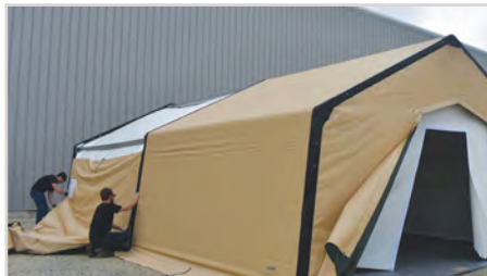
Shelter body panel installation
