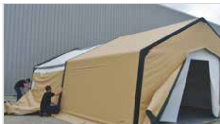
Shelter body panel installation
