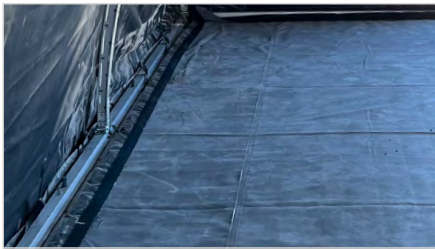
KEDER TRACK GROUND BEAMS PROVIDE VECTOR BARRIER
