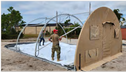
FROM GROUND SET UP NO LADDERS = SAFER
