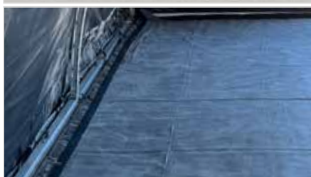
KEDER TRACK GROUND BEAMS PROVIDE VECTOR BARRIER
