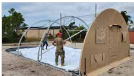
FROM GROUND SET UP NO LADDERS = SAFER
