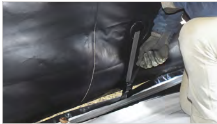
FABRIC TENSION VIA CAM BUCKLES MAXIMIZES FABRIC LONGEVITY
