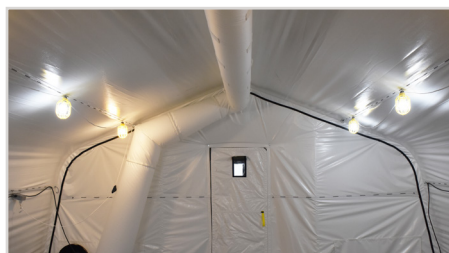
Plenum, lighting, and power receptacles
