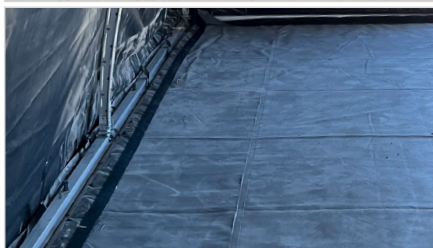
KEDER TRACK GROUND BEAMS PROVIDE VECTOR BARRIER
