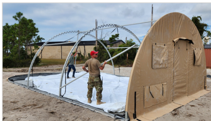
FROM GROUND SET UP NO LADDERS = SAFER
