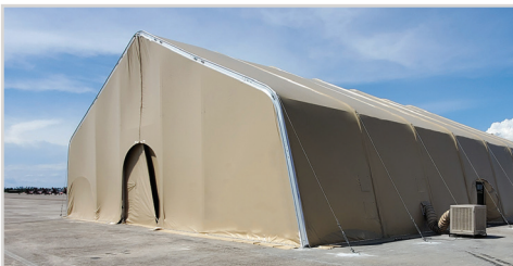
Gable end walls provide supports for personnel doors and entry ways
