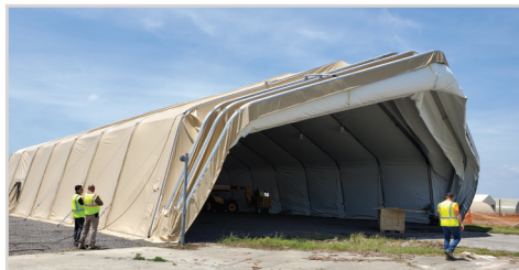
Tri-lid doors allow for maximum clearance when entering the shelter
