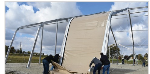
Keder fabric panels install quickly and easily
