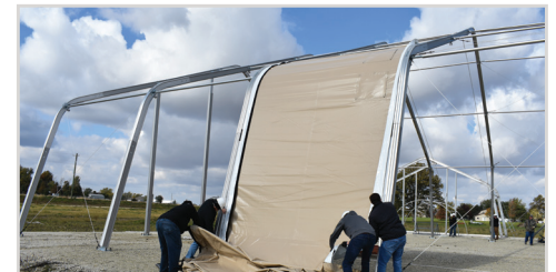
Keder fabric panels install quickly and easily
