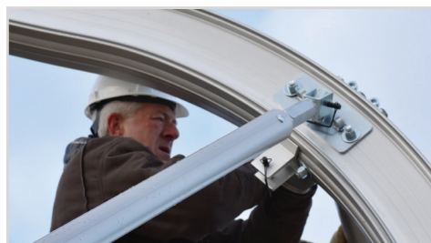
Locking purlins provide enhanced stability across the shelter
